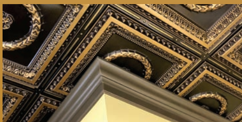
Finish with crown molding
